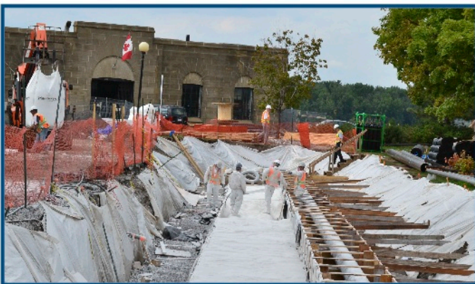
Gilsulate was determined to be more cost effective & efficient than PIP
