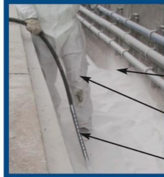
NARROW TRENCH REDUCES EXCAVATION. 24" CWSR. OUTSIDE CFUD THICKNESSES 6" PIPE SPACING 6".
