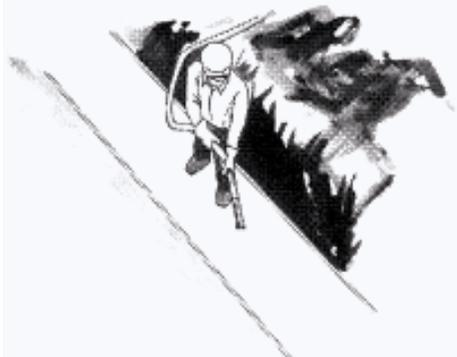
7. Add additional layers of **GILSULATE® 500XR** and consolidate to specified thickness and density. A rod-type concrete vibrator with a 1½" or smaller diameter head is the best and quickest means of consolidating **GILSULATE® 500XR**. Insert the head of the vibrator horizontally and pull along slowly. Larger pipes require consolidation in two or more lifts of material.
