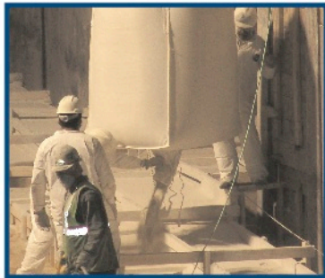
Gilsulate flowing out of its Mega Bag
